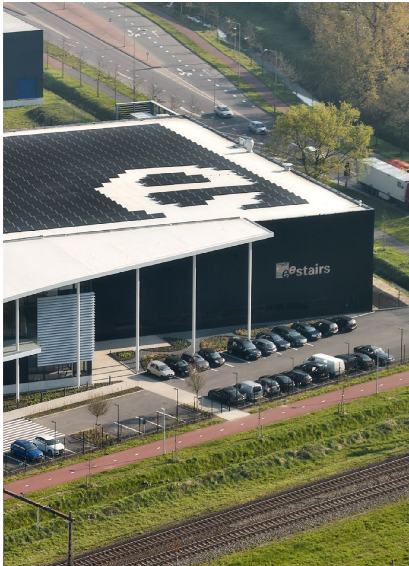
Our BREEAM Outstanding HQ Powered by 600 solar panels
